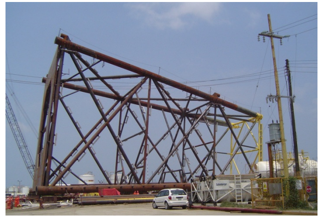
Figure 7. Tetrapod structure at Cobos marine terminal.
