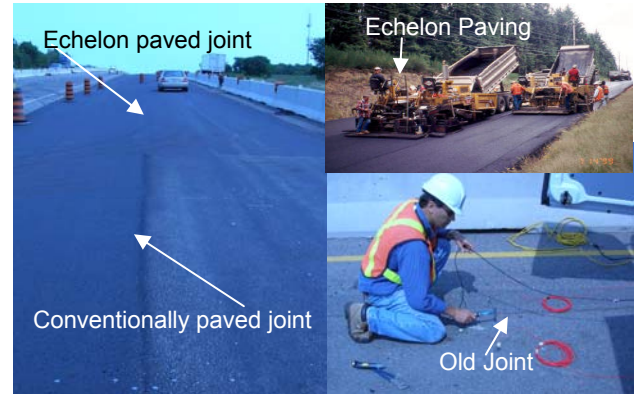
Figure 5. NDT testing of longitudinal joints using seismic waves on Hwy 401
