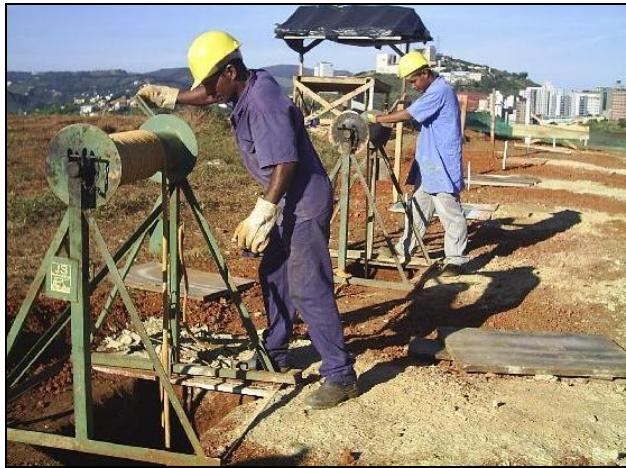
Figure 8. Simultaneously big rectangular excavation (São Paulo, Brazil).
