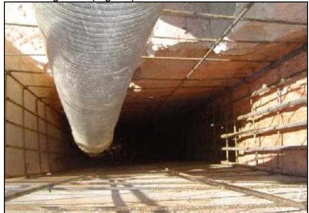
Figure 14. Full section big rectangular concreting (Belo Horizonte, Brazil).
