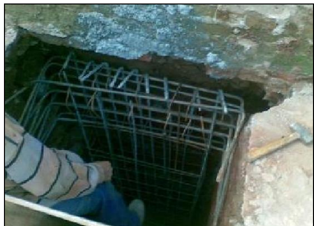
Figure 15. Folded bars in the distribution effort beam (Belo Horizonte, Brazil).
