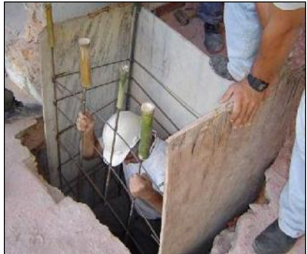
Figure 10. Worker going into the excavation (Belo Horizonte, Brazil).
