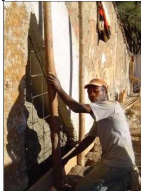
Figure 17. Supplementary curtain implementation (Belo Horizonte, Brazil)
