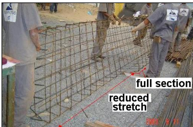
Figure 9. The reinforcing steel prepared outside the shaft (Belo Horizonte, Brazil).
