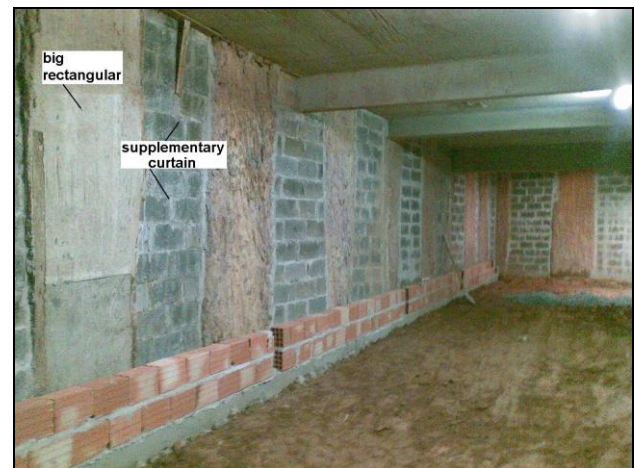
Figure 18. Supplementary curtain using concrete block (Belo Horizonte, Brazil)
