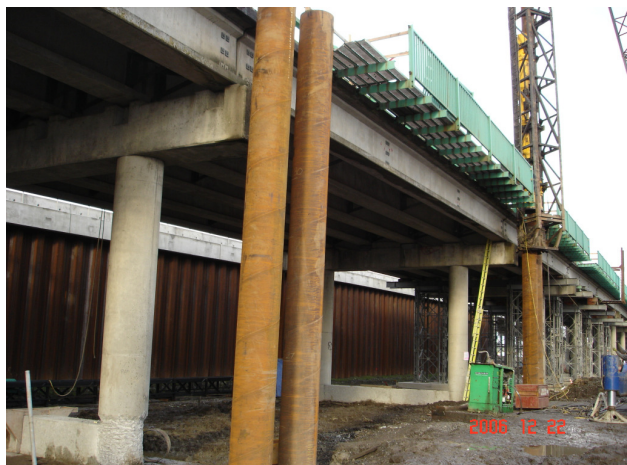
Figure 19 Permanent bridge retrofit including new pile caps and steel pipe piles
