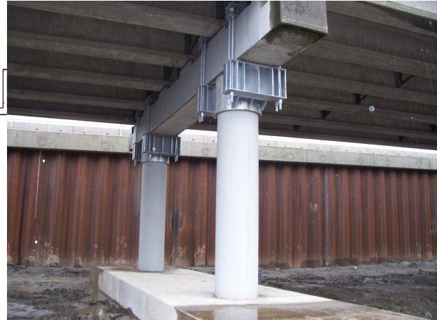
Figure 21. Bent after permanent retrofit (looking west)
