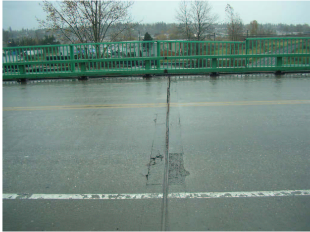
Figure 8. Uneven displacement of expansion joint at Pier 8, and handrail pulled apart at the east side (far side)
