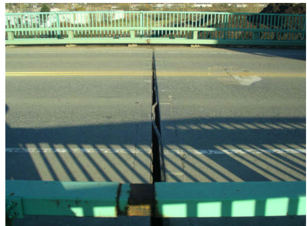
Figure 7. Uneven displacement of expansion joint at Pier 6, and traffic rail pulled apart at the west side (foreground)
