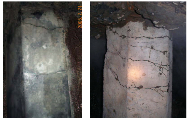
Figure 10. Cracks in precast piles at Pier 5 and Pier 6 on the west side
