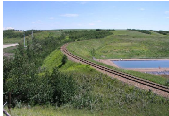
Figure 2. CPR embankment in area of crossing.
