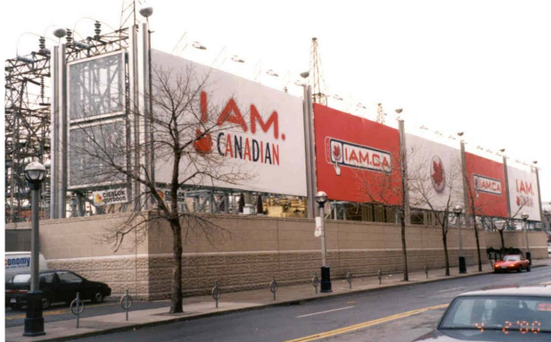
Figure 12. Billboards supported using helical piles
