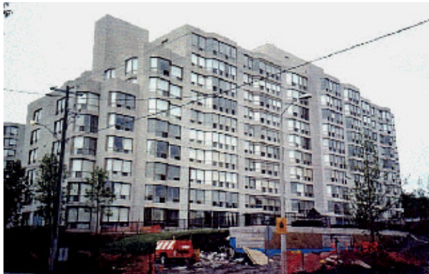
Figure 2. Photograph of 11-storey residential building
