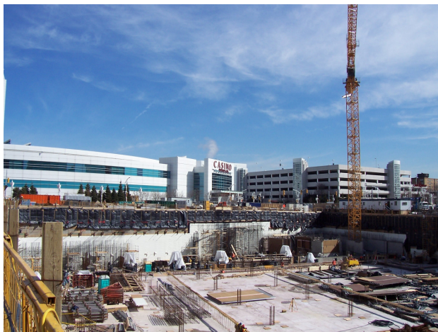
Figure 9. Project during construction
