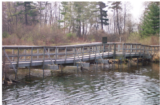
Figure 11. Boardwalk supported using helical piles
