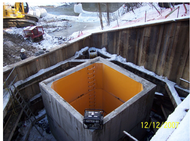
Figure 8. Fox Hollow sanitary trunk sewer manhole
