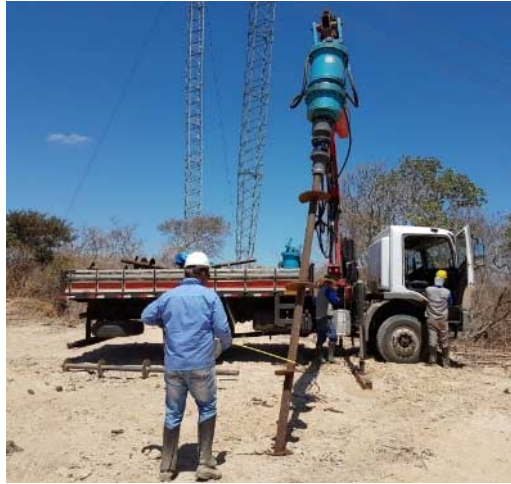
Figure 1. Helical pile installation in a Brazilian transmission line.
