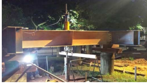
Figure 6. Load test set-up.
