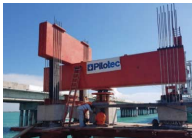
Figure 6. Reaction frame arrangements on type 1 abutment.
