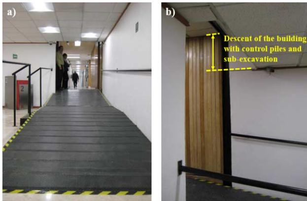
**Figure 8.** Current condition of one of the corridors communicating with an adjacent building (November 2018): a) front view and b) side view.
