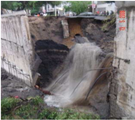
Figure 7. Fault on the diaphragm wall and post-tensioned anchors.
