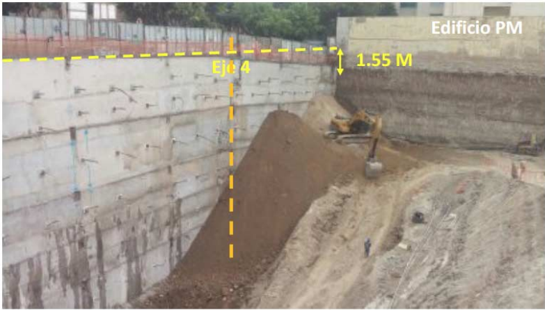
Figure 9. Twisted shotcrete wall; the surcharge of stabilizing material is appreciated.
