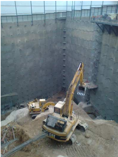
Figure 1. 54.5 m excavation.
