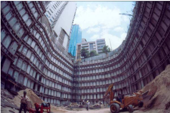
Figure 5. Precast diaphragm wall with secondary beams and anchors.
