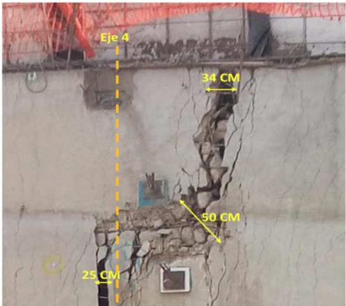
Figure 10. Detail of the shotcrete wall cracks due lo sliding and twisting.
