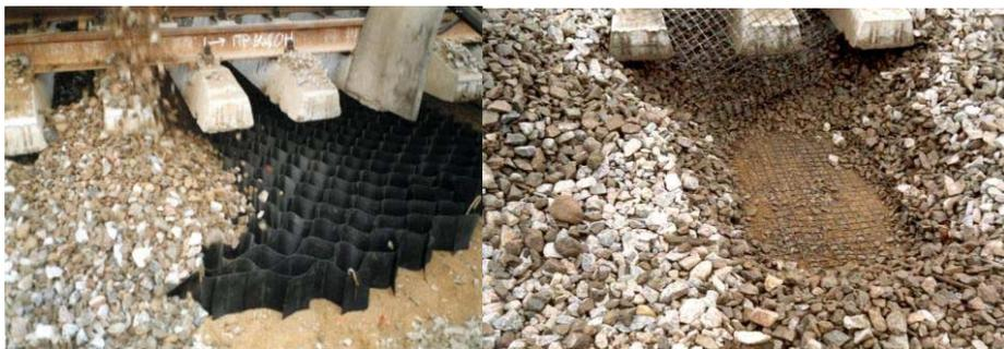
**Figure 1.** Laying of geocells and two geogrid layers.
