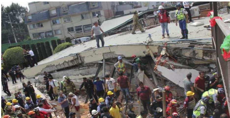
Figure 4. Collapse of school in the 2017 Puebla-Morelos earthquake (Photo by Carlos Cisneros/AP).
