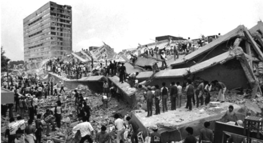
Figure 3. Collapse of residential multistory building in the 1985 Michoacán earthquake [13, 19].
