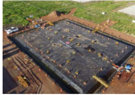
(b) Airtight membrane technology (Start: May 10, 2017 - End: May 7, 2018)
