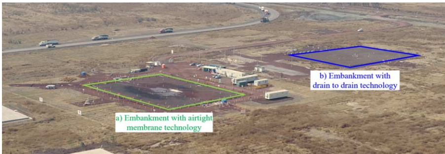
Figure 1. Test embankments with simple preload, PVDs and vacuum: (a) drain-to-drain and (b) with an airtight membrane at the NAICM site (photo courtesy of E. Botero, 2018).
