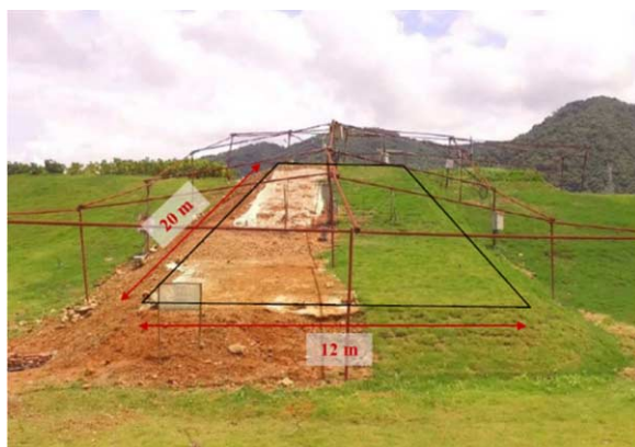
Figure 2. Front view of the Xiaping landfill site in Shenzhen, China.
