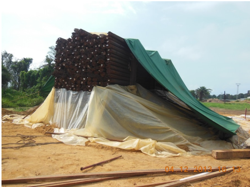
Figure 3. Kentledge (reinforcing steel stacked to 500 tons) setup completed
