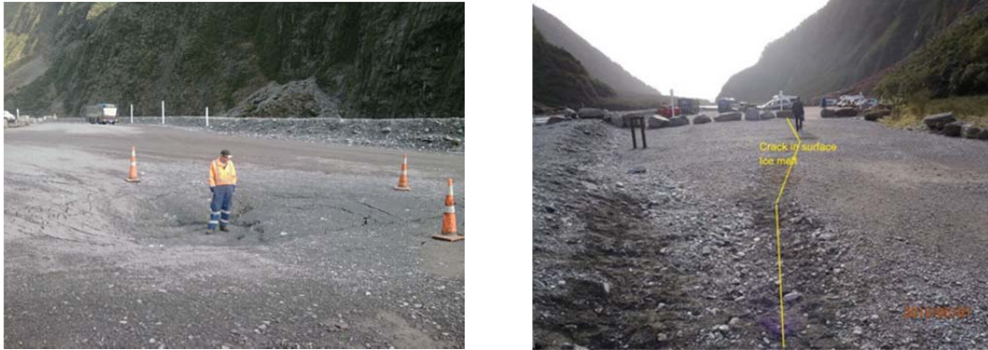
Figure 4. Photographs of subsidence
