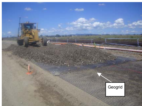
Figure 9. Installation of geogrid under the ballast at Singleton, NSW
