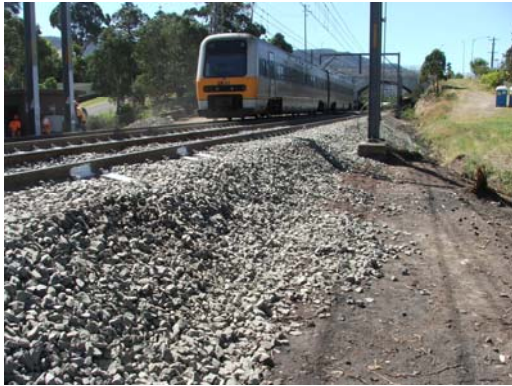
Figure 9. Instrumented track at Bulli
