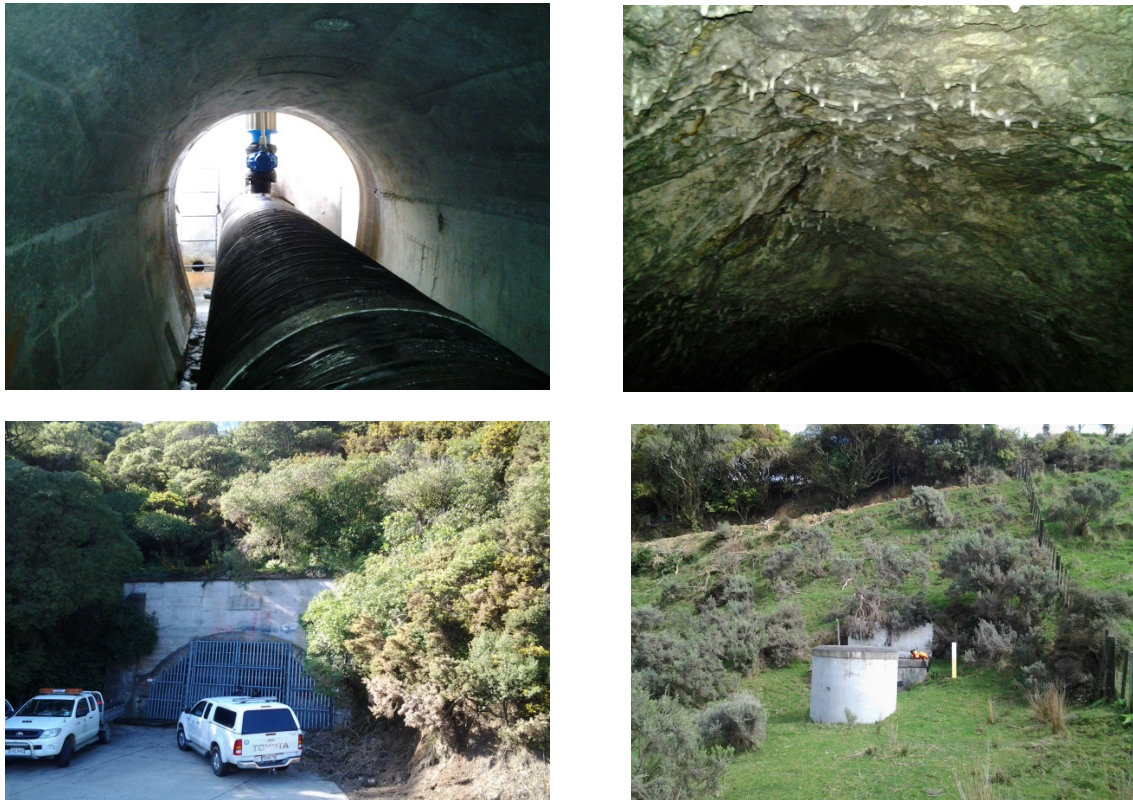
Figure 2. Typical lined tunnel, roof of an unlined tunnel, and tunnel portals
