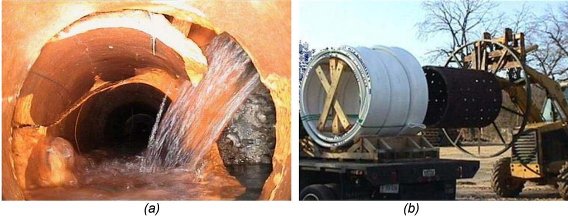
Figure 1. (a) Example of damaged sewer pipe as a result of 2011 Christchurch Earthquake (ProjectMax 2012); (b) Coil of AM-Liner (American Pipe & Plastics Inc 2005)
