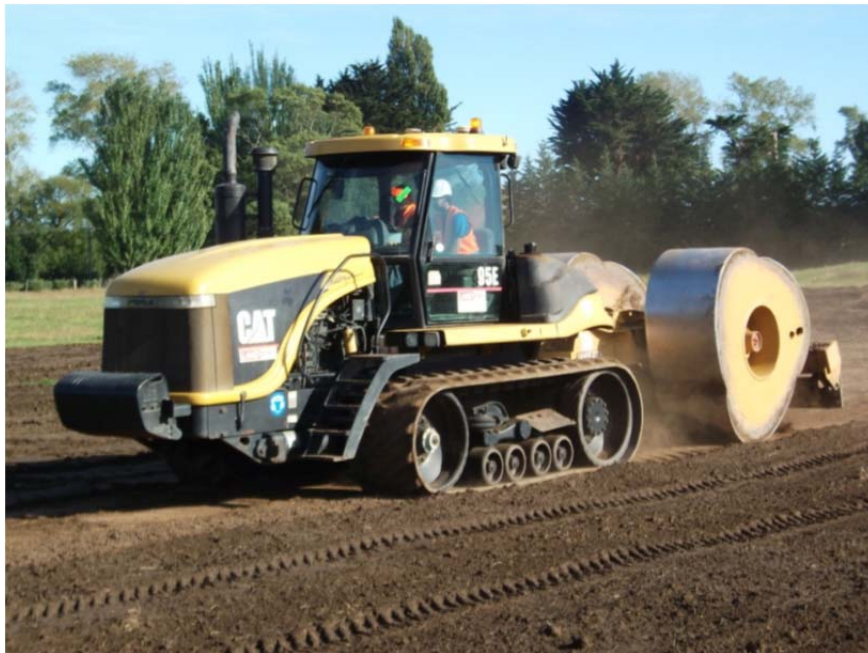
Figure 3. Impact compactor working at the Prestons Subdivision
