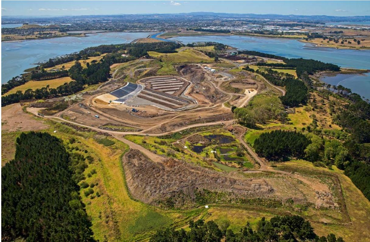
*Figure 1. Aerial photo of the site in early 2014, showing the containment facility haul roads, embankment, and liner under construction (centre of photo), and Manukau Harbour surrounding the Island. Photo credit: Watercare Services Ltd.*
