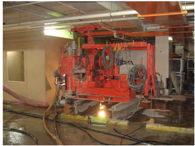
Figure 3. Installation of jet grouting columns in the Art Gallery basement
