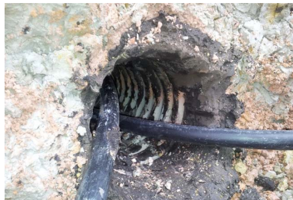
Figure 3. Grooved auger hole
