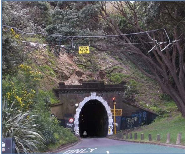
Figure 1. The current eastern portal with wingwalls either side
