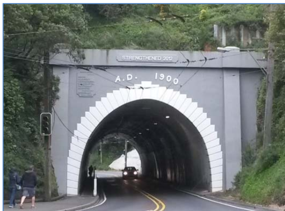
Figure 4. Portal post strengthening
