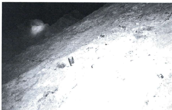
Figure 6. Roof Collapse in Gallery C showing sheared rock bolts in roof collapse debris
