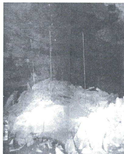
Figure 3. Roof Collapse in Gallery A showing portion of roof collapse debris and protruding rock bolts.
