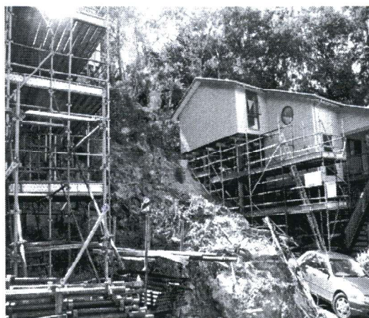
Figure 1. House on Failed Slope Showing Scaffolding Support and Reinforced Piers
