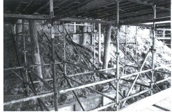
Figure 3. House on Failed Slope Showing Scaffolding Support and Rotated Piers
