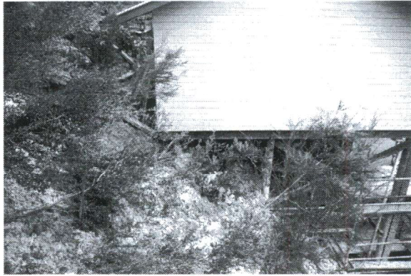
Figure 2. House on Failed Slope Showing Rotated Timber Piers
