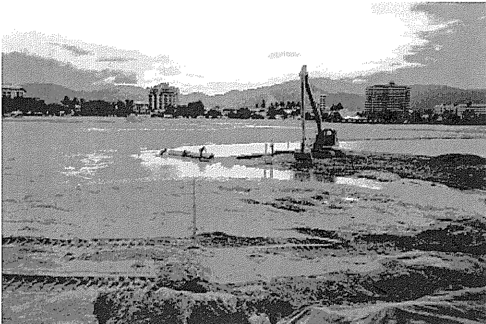
Figure 5. Completing the perimeter of the reinforced fill – note “problems” are contained inside the works.
