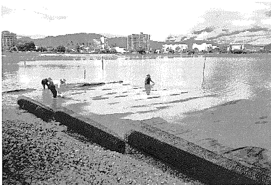
Figure 4. Working underwater – note workman up to his waist in mud when working off the basal layers.
