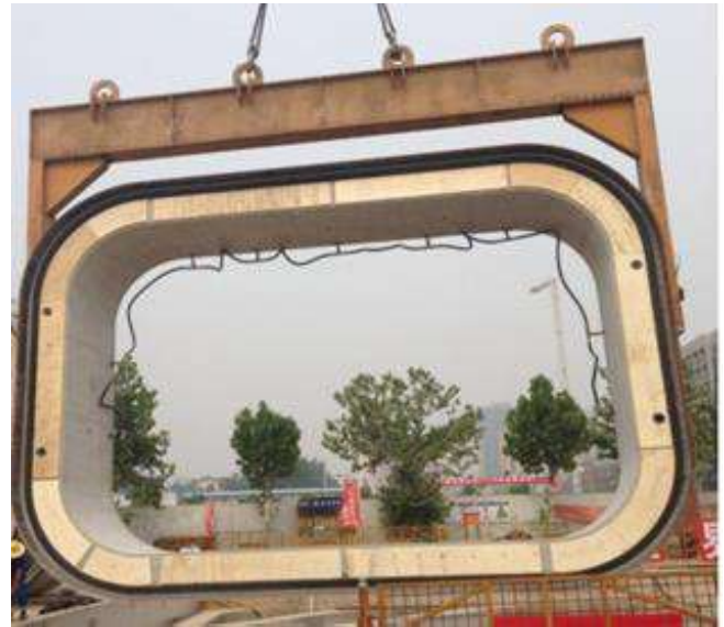
Figure 4 Jacking segment, lifting into the jacking shaft.
