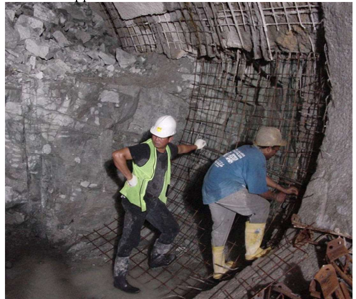
Figure 19 Tunnel excavation.
