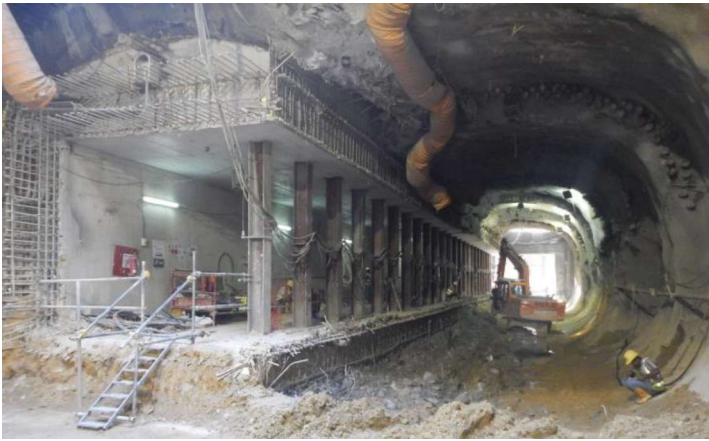
Figure 17 Excavation completed. Permanent works completed on the left side.
