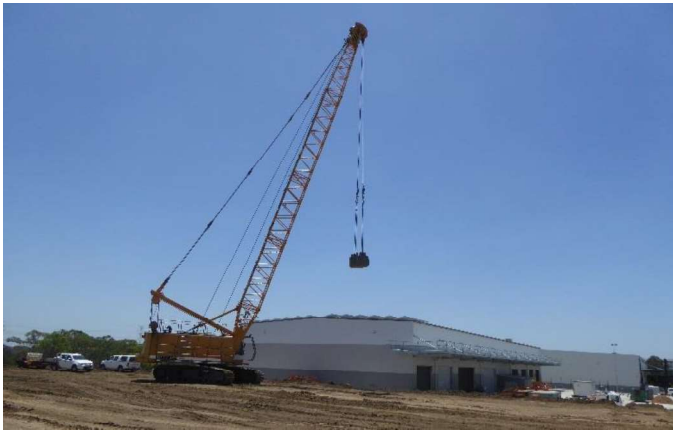
Figure 4. Application of dynamic compaction approximately 25 m away from an existing building
