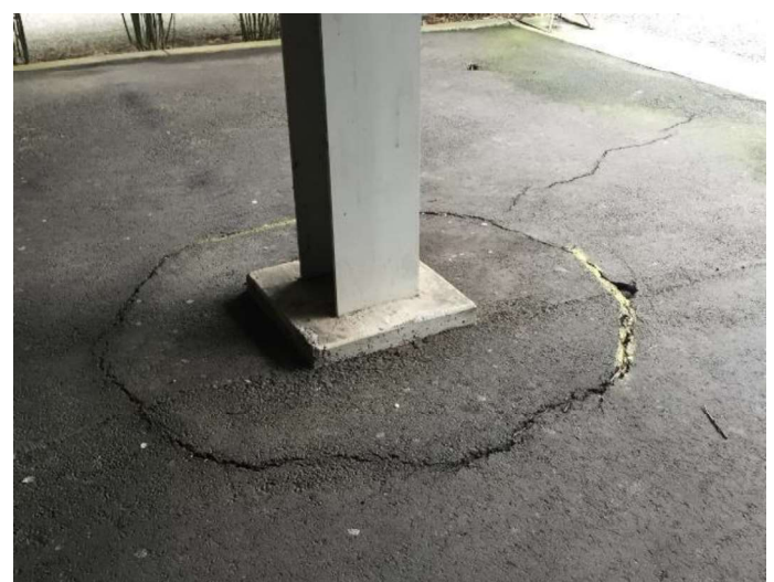
Figure 4. Differential settlement between piled footings (CP6 West) and the surrounding asphalt pavement.
