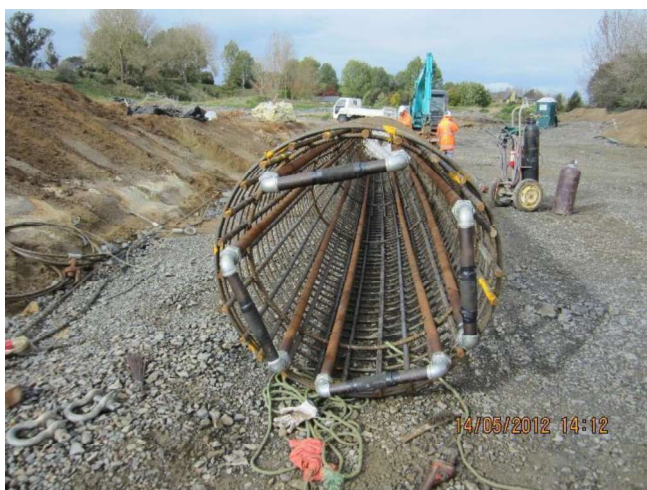
Figure 2. Grout tube arrangement Waikato River Bridge
