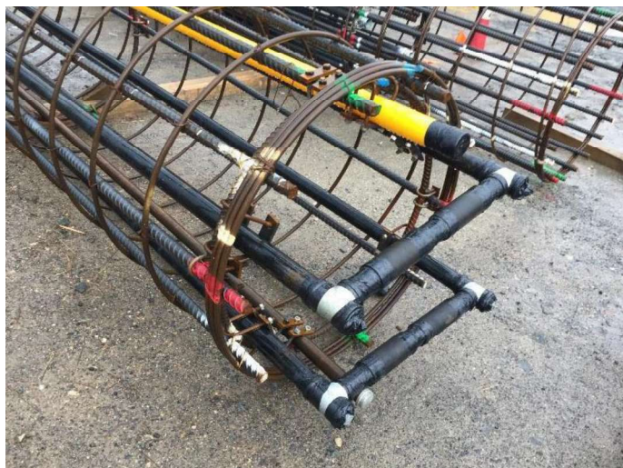
Figure 4. Grout tube arrangement Mangaonua Stream Bridge
