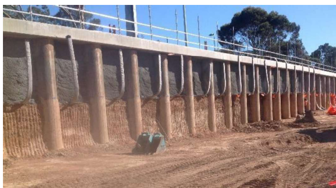
Figure 7. Shotcrete infill with vertical strip drains
