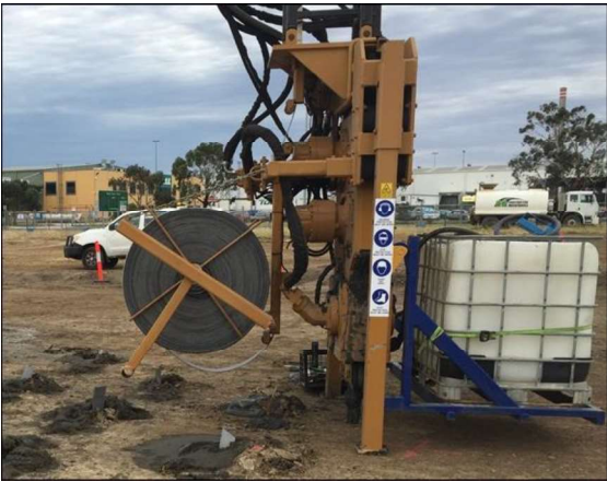
Figure 5 – Wick drain installation
