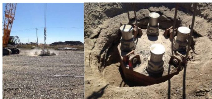
Figure 6. Pounding in progress (L), Crater and pounder (R)
