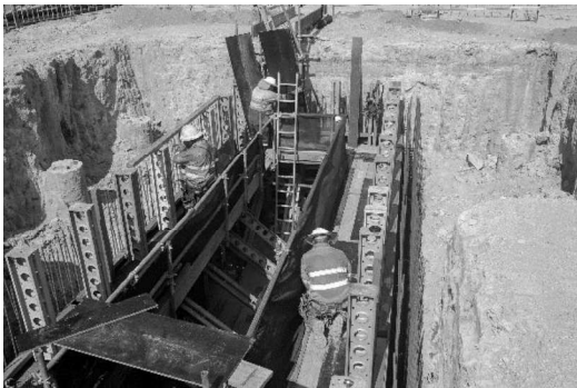
Figures 10. Construction of RFSP
