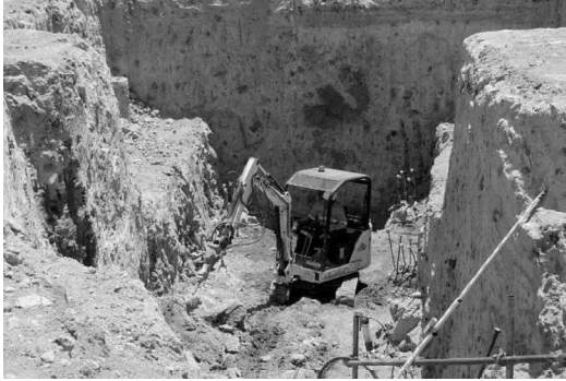
Figures 9. Excavation at RFSP
