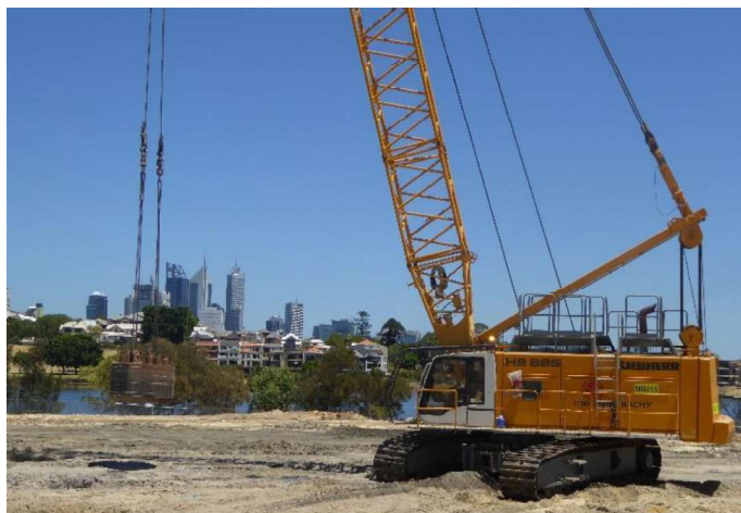
Figure 5. Application of dynamic compaction at Optus Stadium
