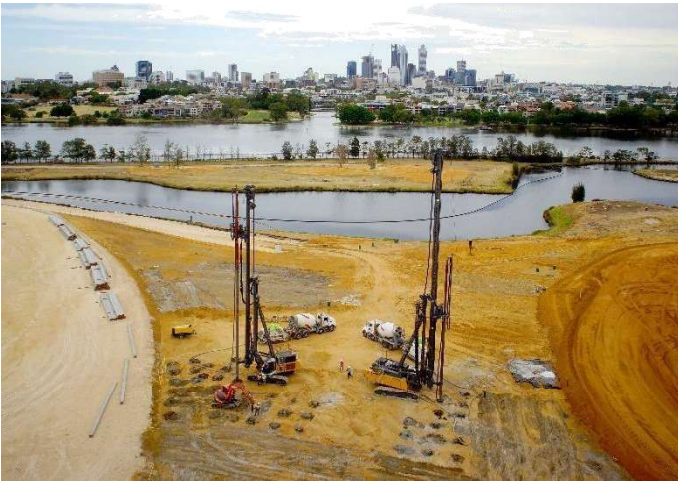
Figure 4. Installation of CMCs at Optus Stadium
