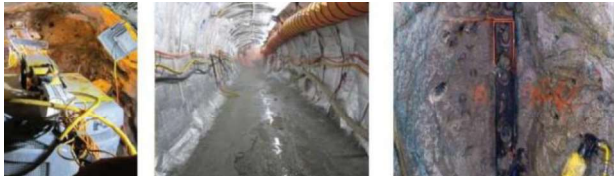
Figure 8. Gallery excavation (after Polycarpe et al. 2012)
