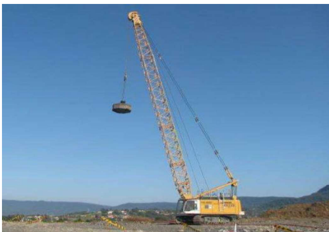
Figure 1. Deep Dynamic Compaction equipment.
