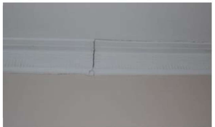
b) most severe damage observed in internal linings.
