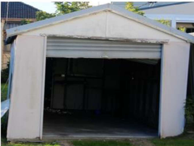
b) tilts in the garage (see slab contours in Figure 2).
