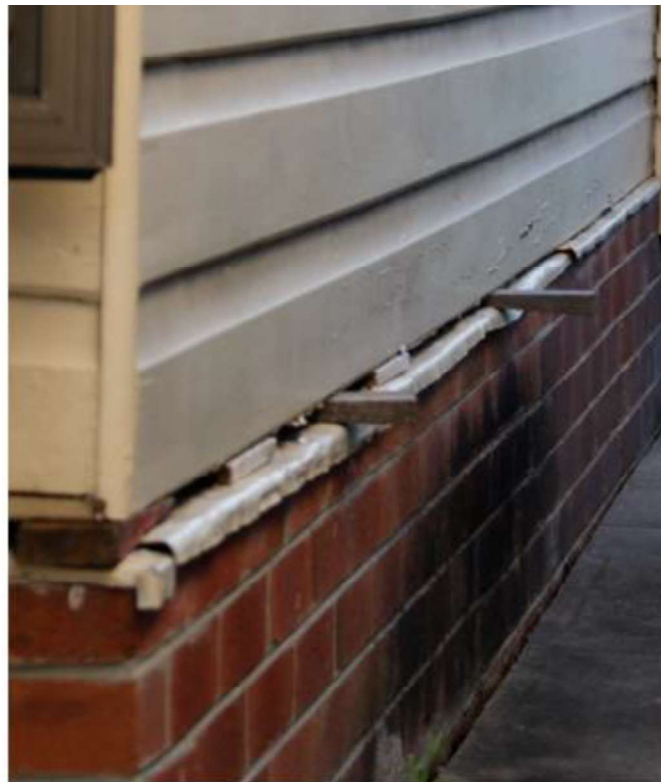
a) packing of gaps between house and support walls
