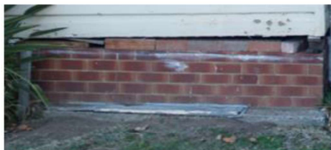
b) severe settlement of support walls
