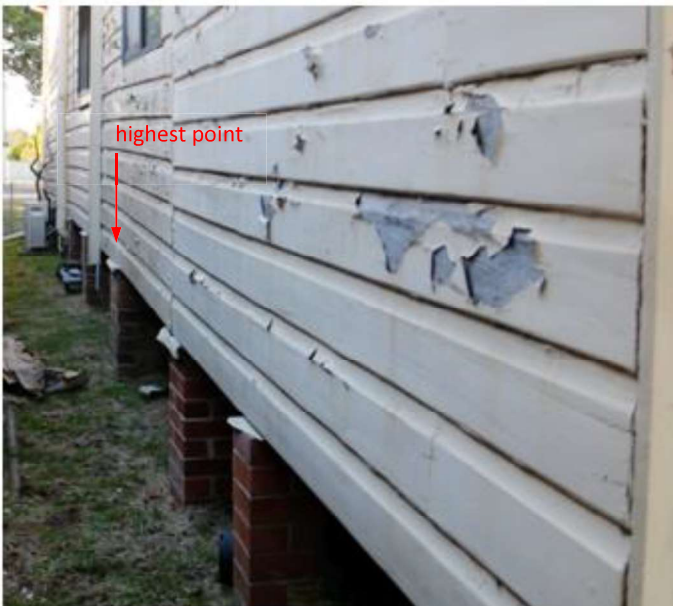
a) curvature of weatherboards along the side of the house. (wall C-D in Figure 4b)
