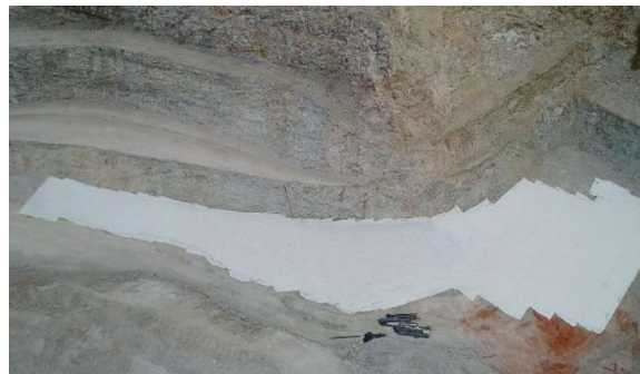
Figure 5. First layer of geofabric completed.
