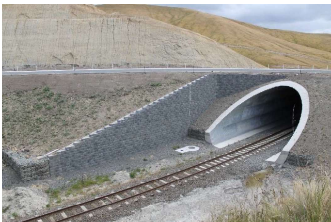
Figure 6. Keystone TW3 west wall at Dashwood completed
