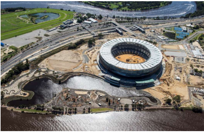
Figure 1. Optus Stadium during construction, looking east.
