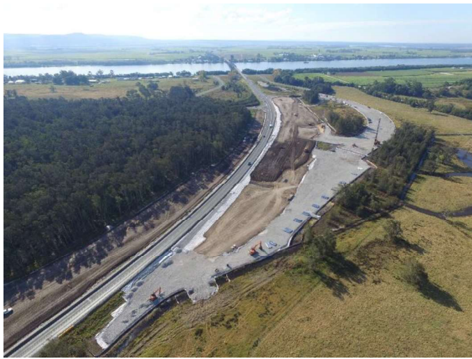
Figure 2. Early works construction at Yamba interchange (2017)
