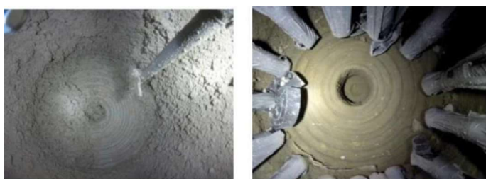
Figure 7: Photographs of pile base before and after being cleaned.
