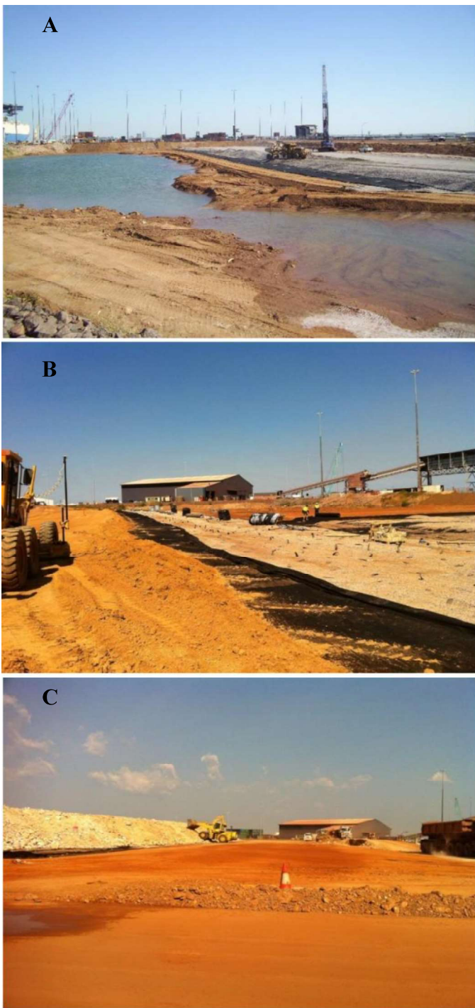
Figure 5: PVD Installation (A), ongoing earthworks (B) and placement of surcharge (C)
