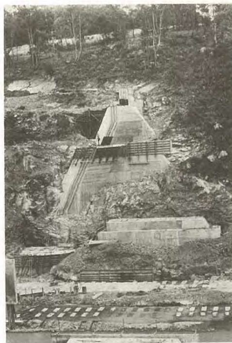
Fig. 5 - Left abutment - note buttress foundation supporting base of cut.
