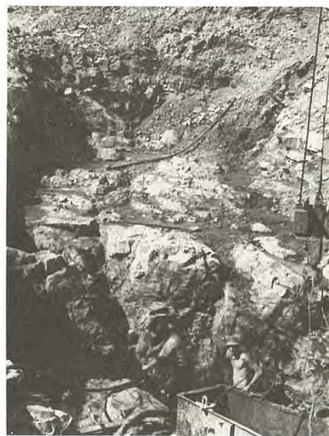
Fig. 3 - Clay seams and altered fractured basalt in fault trench.
