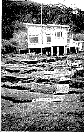
Fig. 5 Coledale Heights, Illawarra - Note closely spaced tension cracks within failed area
