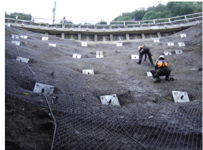
Figure 1: Soil nailing for strengthening Ngaio Gorge Road
