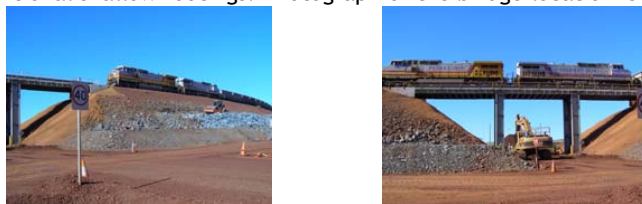
Figure 1: Photographs of the bridge duplication location
